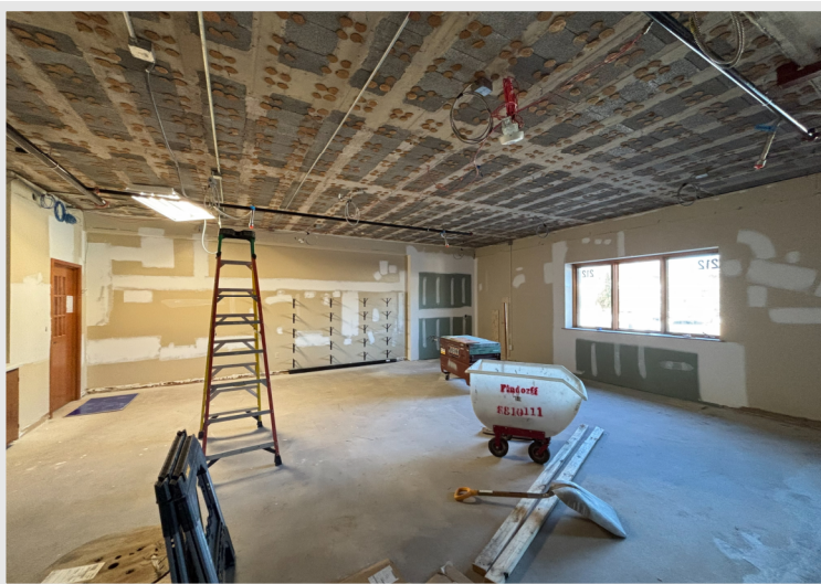
Drywall taping/finishing in progress in the Second-Floor 3 rd Grade Classroom bringing the new and existing walls to life!
