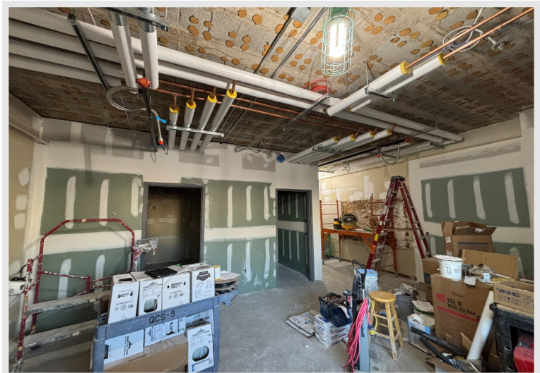
Drywall taping/finishing nearly complete in the First-Floor Speech Offices in preparation for painting closely behind!
