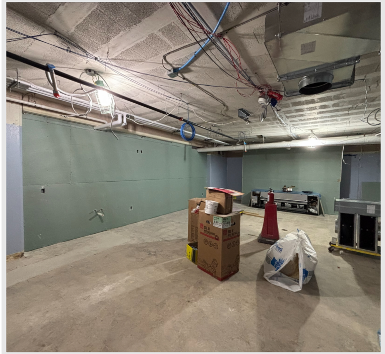
Drywall installation complete with the new unit ventilator set in the Lower-Level OT/PT space! Taping/finishing to follow shortly...
